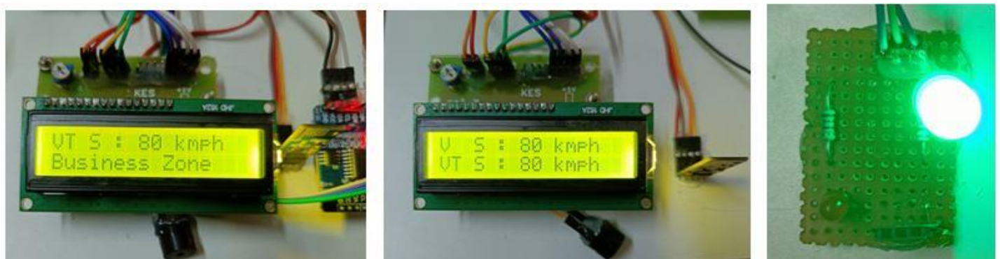
Figure 7 : Vehicle speed is controlled and alerting system became normal
