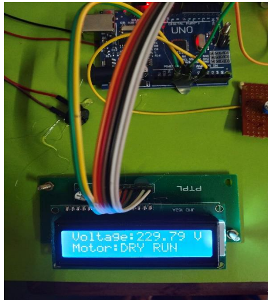
Fig 3: when the system is in normal condition during dry run
